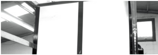
Reinforced front wall and corner posts
