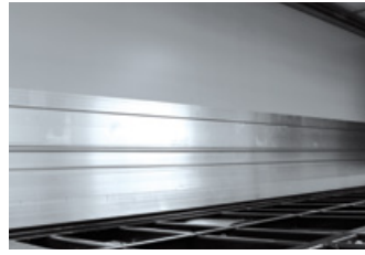
Upper wall made of aluminium honeycomb panel, lower wall made of aluminium profiles
